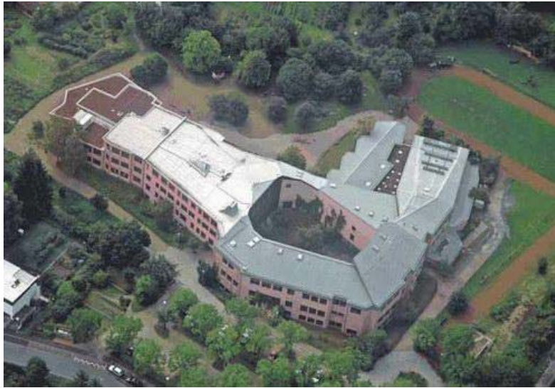
Figure 4. Aerial view of Freie Waldorfschule, Darmstadt, Germany
